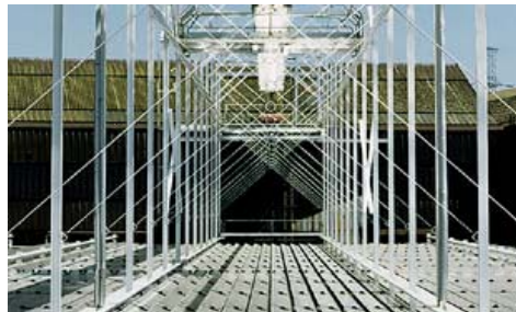
Figure 1: Prototype of the Fresnel collector (2,500 m 2 ) erected by the company Solarmundo, Belgium. On the bottom of the image: the Fresnel mirrors, on top: the collector tube covered by a thermally insulated secondary mirror (source: Solarmundo).
