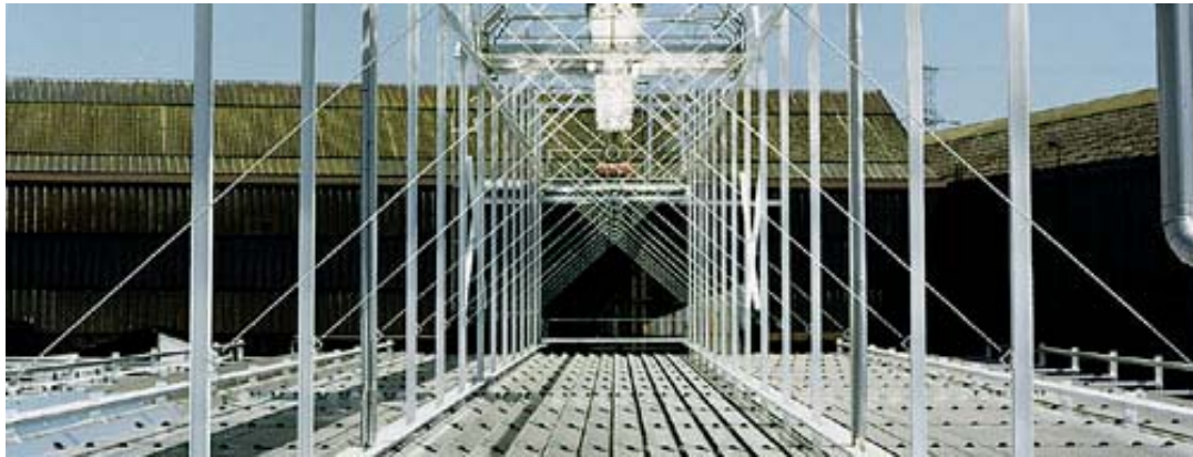
Figure 1.2: Prototype of the Fresnel collector at Liege (Belgium) developed by Solarmundo
