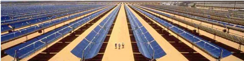
Rows of parabolic troughs swivelling to track the sun
