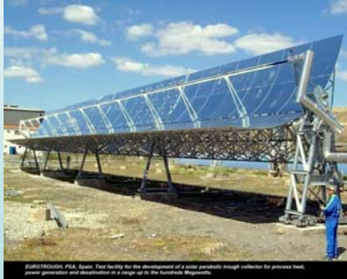
Eurotherm, PSA, Spain. Test facility for the development of a solar parabolic trough collector for process heat, power generation and desalination in a range up to the hundreds Megawatts.
